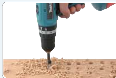
Drilled through holes in 60mm thick Lauan with \phi 15 Auger bit.
