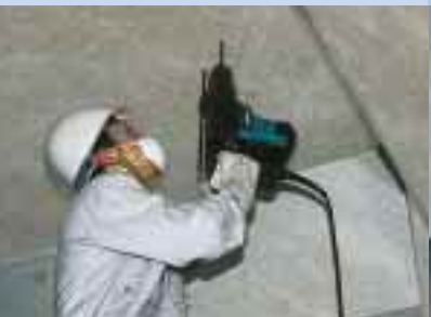
Masonry drilling with carbide tipped bits
