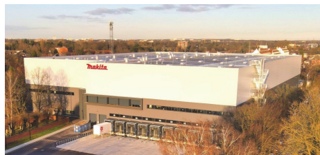
Logistics Warehouse at Our Germany Plant
