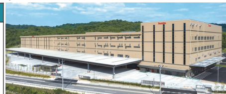
Okayama Distribution Center (with branch/sales office)
