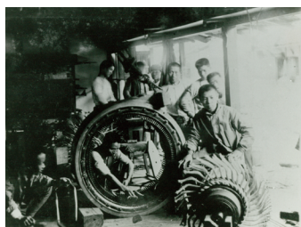
Repairing electrical machinery
